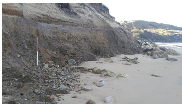
Broughton Bay cliff erosion
